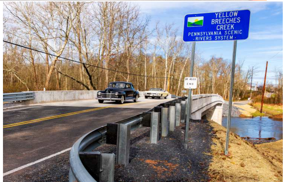
JV308: The new Andersontown Road bridge, pictured right, over the Yellow Breeches Creek replaced a single lane bridge, pictured above, that was built in 1930 with an open steel grate deck. The old bridge was also posted for weight limits. Work performed by Walsh Construction
