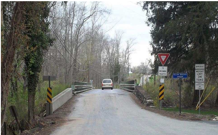
JV308: The new Andersontown Road bridge, pictured right, over the Yellow Breeches Creek replaced a single lane bridge, pictured above, that was built in 1930 with an open steel grate deck. The old bridge was also posted for weight limits. Work performed by Walsh Construction
