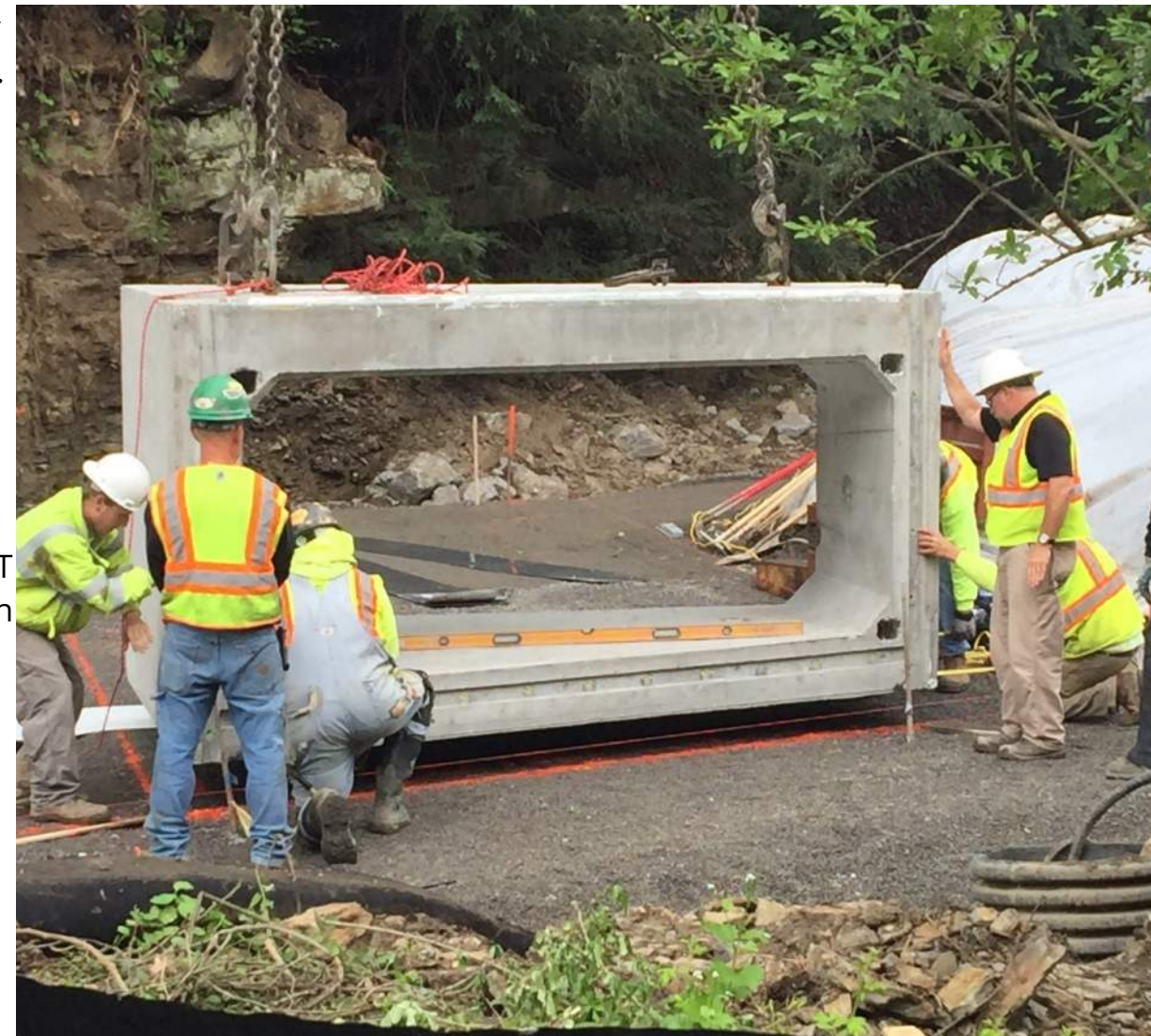
It's a skillful job setting the first box culvert section at JV-413 in Indiana Township, Allegheny County (PennDOT District 11).
